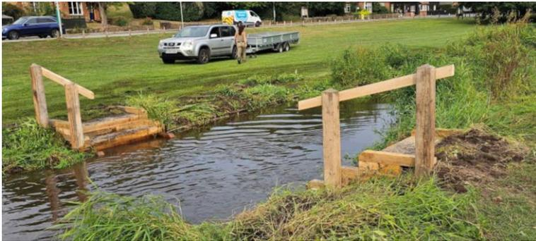
To reduce the rate of bank erosion we installed some oak steps with a handrail to make access in and out the stream easier.
